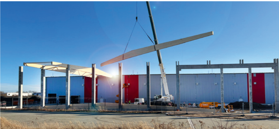
3 months after the ground-breaking ceremony at B&O Holzbau GmbH, the silhouette of the company's new Hall No. 3 is clearly visible. The transportation and installation of the glued timber trusses, which are necessary for the roof construction, has been extremely challenging. Each one of the 15 custom-made products is approx. 40m long, 2m high and 27cm wide.
